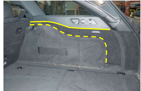
Carpet finishes at a plastic sill that follows the shape of the side
